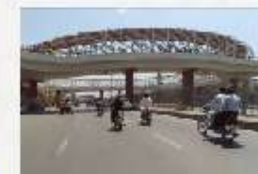
NEAR TO MAIN FEROZPUR ROAD
